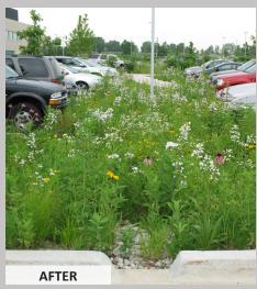
The implementation of green infrastructure is a best management practice intended mainly to filter pollutants from stormwater. Common applications are bioswales, rain gardens, and bioinfiltration basins. They often include engineered soils, under drain systems and native plants.
