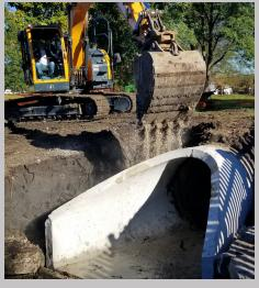
Gray infrastructure includes the use of underdrain pipe systems, fixing or modifying concrete pipe flared end sections, creating curb cuts to allow proper drainage, the use of cisterns or rainwater harvesting systems, and the installation or management of water control structures.
